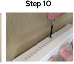
Replace retainer screw and tighten
